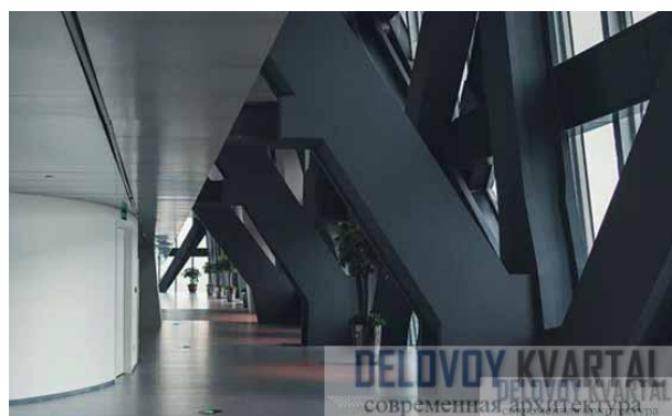
Fig. 4. Structural elements of the building that make their way through the interiors.
