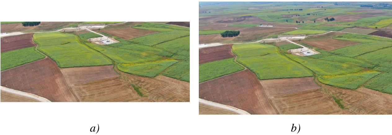
Fig. 1. Photographs of the well drilling site of various sizes [2]
