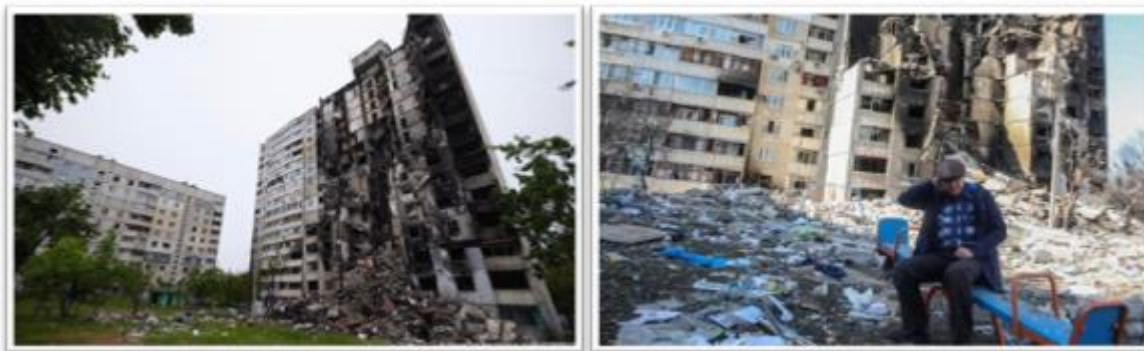
Fig. 1. Destroyed residential buildings in Kharkiv as a result of artillery shelling.
