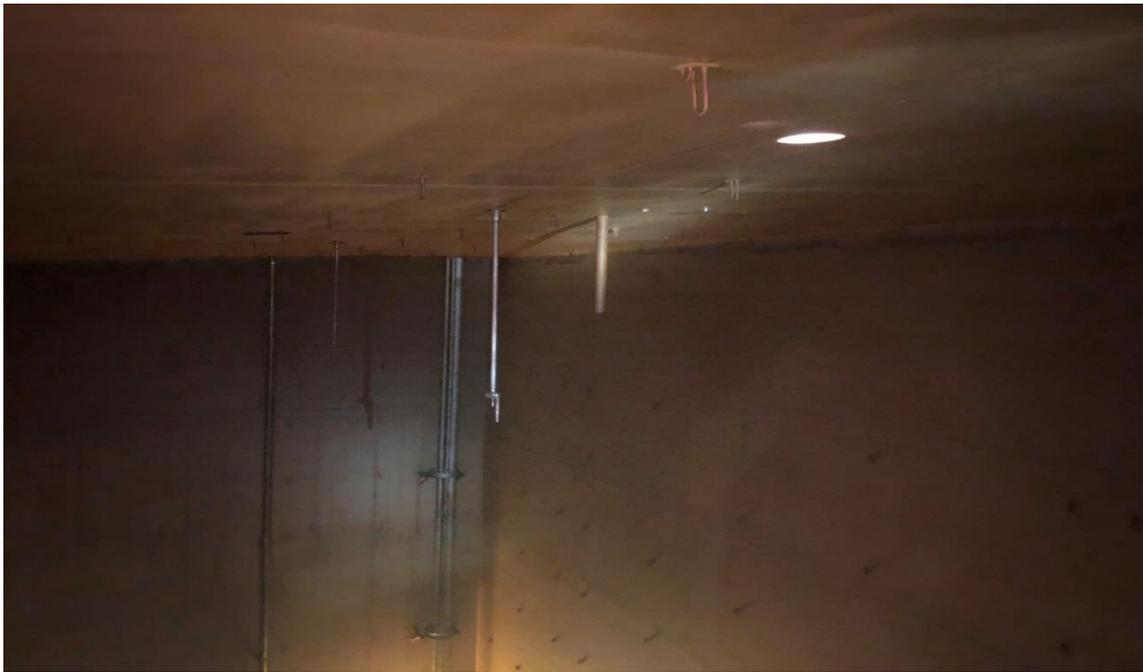
**Photo 1 - Photograph of the cargo tank showing: 95% and 98% fill gauges, tank washer nozzles, pump piping and radar piping for drain level and cargo temperature measurement**
