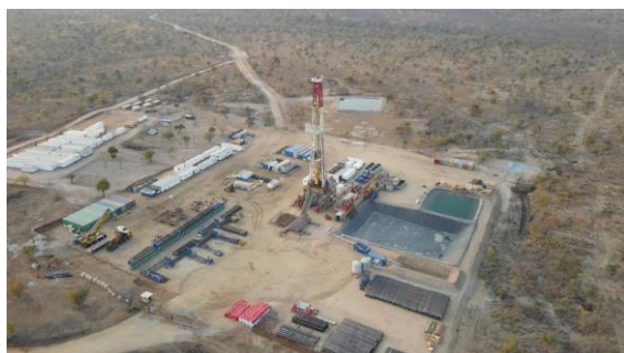
Fig. 2. Exalo Rig 202 at Mukuyu-1 wellsite [1].
