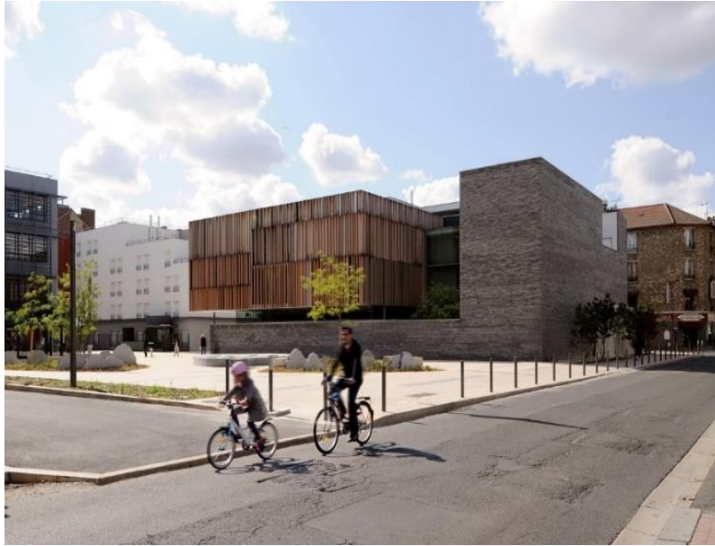
Fig.4 Regional court and industrial tribunal in Montmorency, Val d'Oise, Ile-de-France, France
