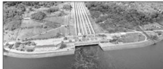
Infrastructural regime facility of HPP, Kyiv, Ukraine
