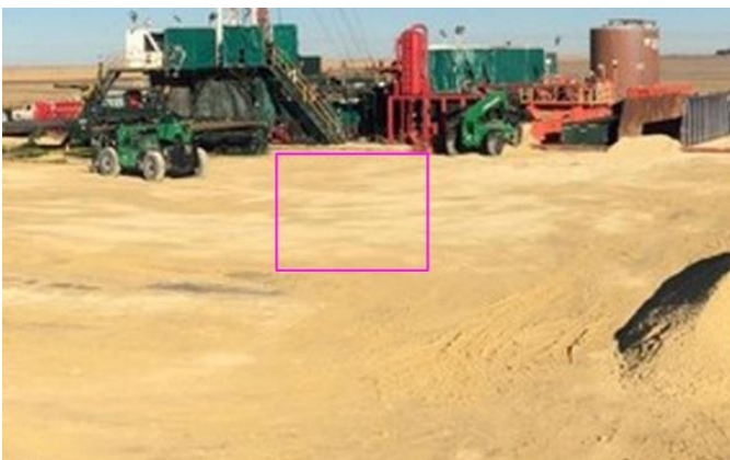
Fig. 1. Photo image of the well drilling site in Nebraska (USA).
