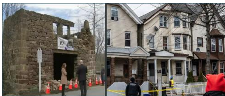
Figure 2. Damage from the earthquake. Left: The historic Col. John Grist Mill at Whitehouse Station had a roof collapse and parts of a wall tumbled onto an adjacent road. Right: Parts of a residence in Newark were temporarily closed after structural damage was found. Sources: 6abc News, The New York Times.
