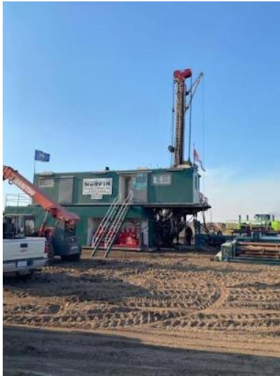
Fig. 3. Photograph of the drilling site of the “Duroche” well.
