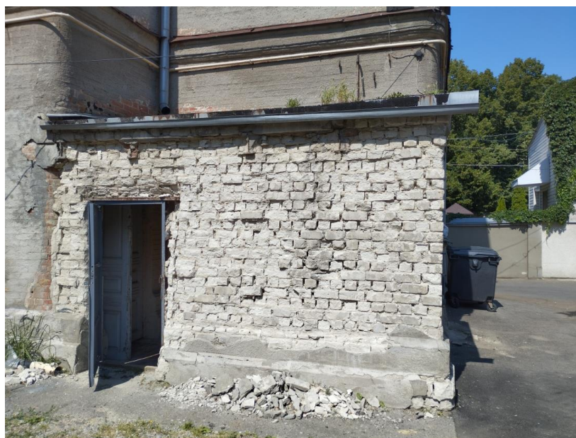
Figure 1. Exterior view of a brick outbuilding
