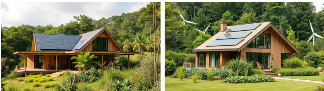
Figure 4. Ecological bamboo houses, project of the company proiectări.md
