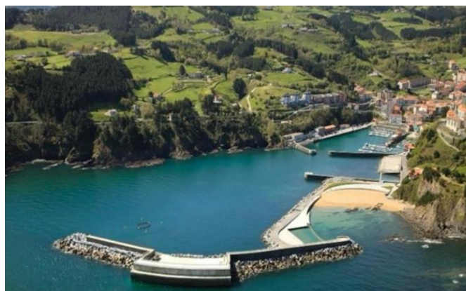
Fig. 2. Picture of the Mutriku Sea Wave Plant
